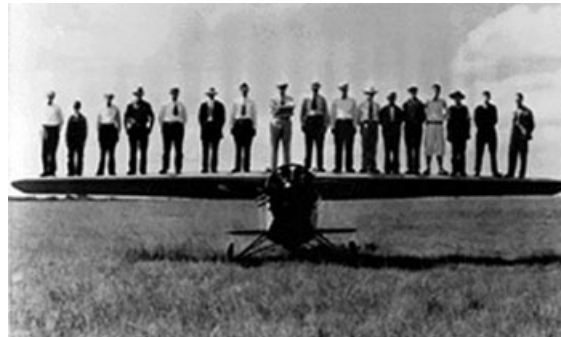
Cessna had some of their employees stand on the wing to show how strong the cantilever wing was.
